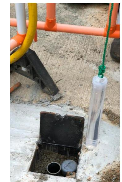
Set-up of Monitoring Well
