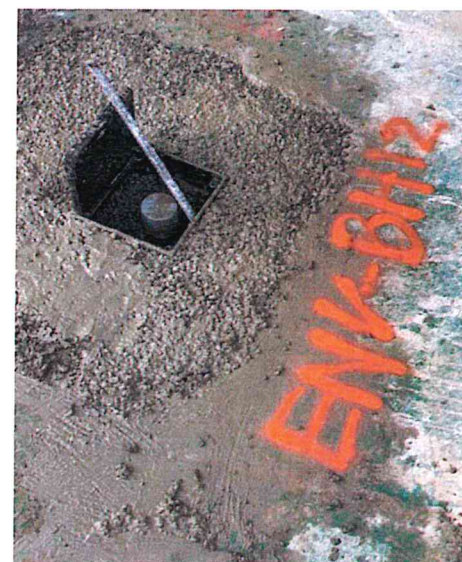
Set-up of Monitoring Well
