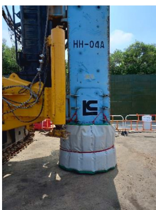
Acoustic material wrapped around the piling head
