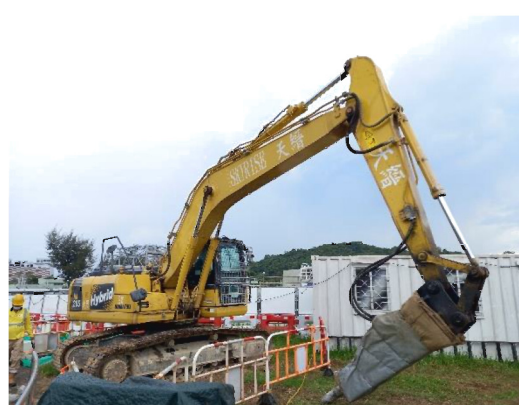
Acoustic material wrapped around to breaker head
