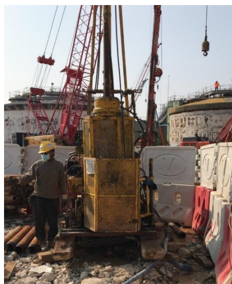
Preparation for Drilling
