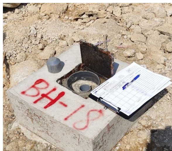
Set-up of Monitoring Well
